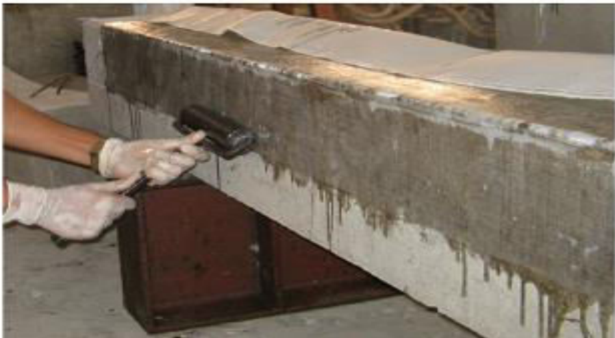
Figure 8: Roller used for removal of air bubbles
