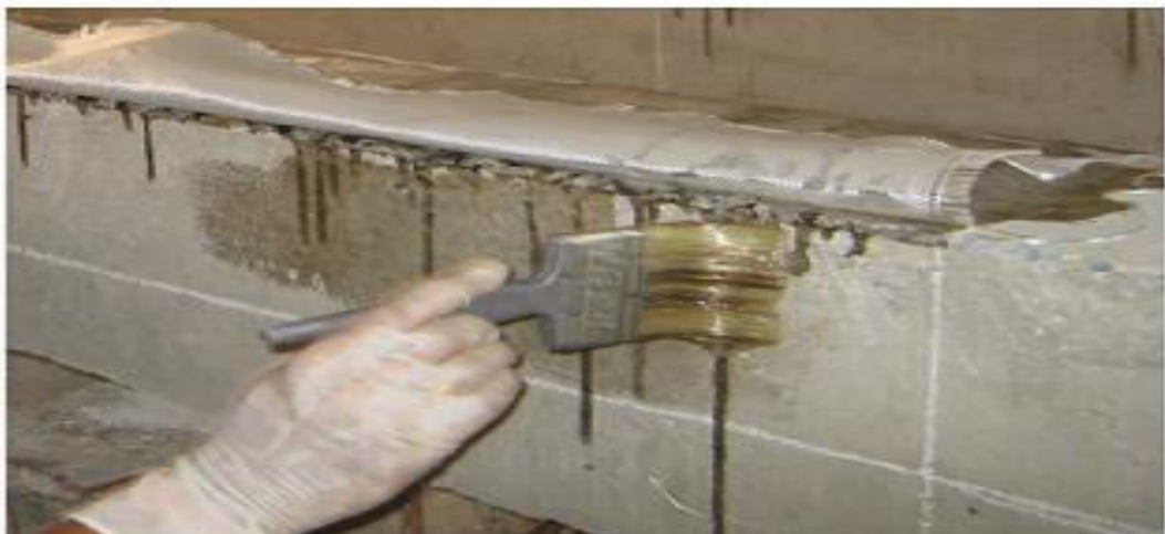
Figure 6: Application of epoxy and hardener on the beam
