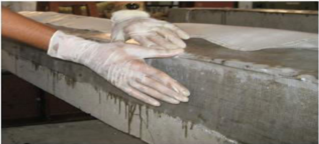
Figure 7: Fixing of GFRP sheet on the beam
